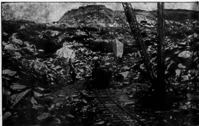
View at the Plant Showing Hand Selection of Rock in the Pit for Transportation to the Crusher.
